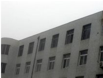
View of the building and its reinforced windows
